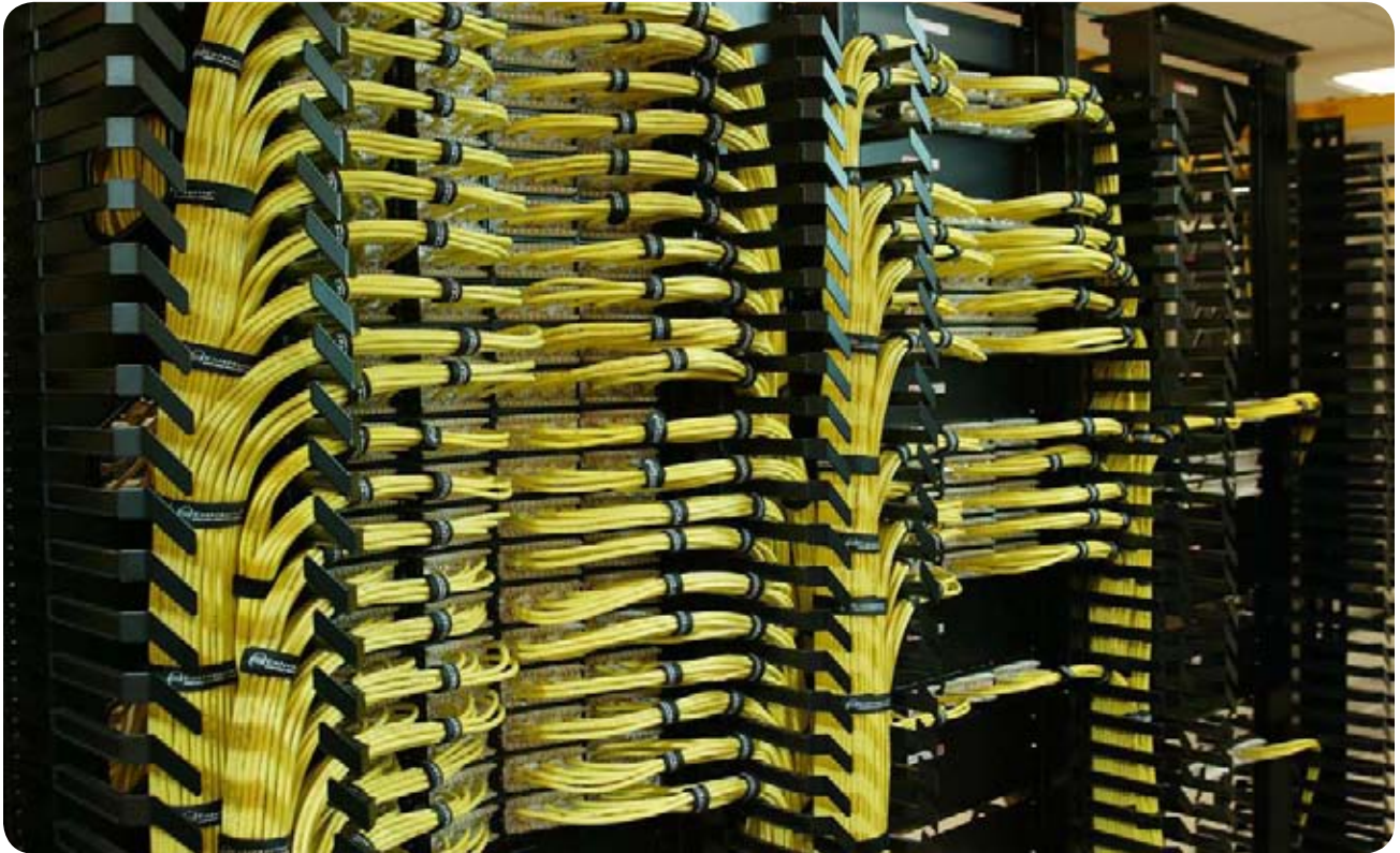
Figure 5. Cable Racks
