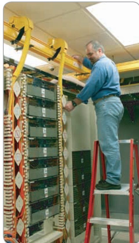
Figure 5. Elements of Cable Management with ADC KRONE Racks
