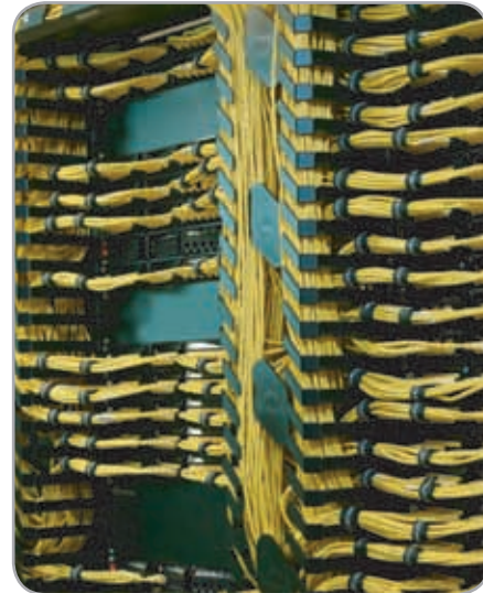
Figure 2. Elements of Cable Management with ADC KRONE Racks
