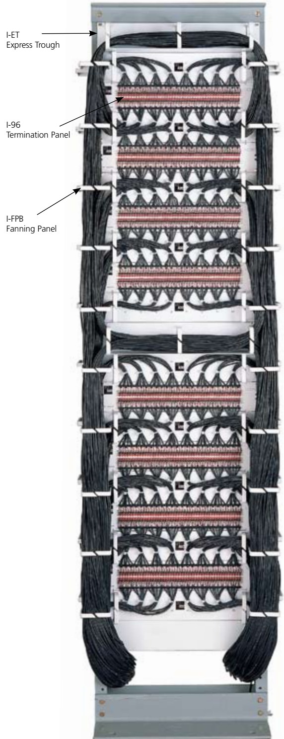
Fully Loaded I-96 Rack-Mount System with Fanning Panels and Express Troughs. Handles 768 balanced audio pairs
