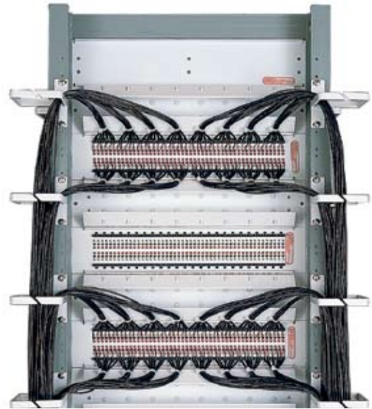
I-96 System (rear view)
