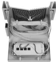
Top Cover Removed (splicing area open)
